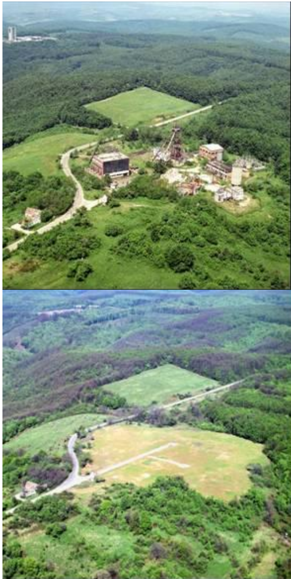
Figure An7.2.3-1: Air shaft IV of the uranium ore mine during operation and after remediation
