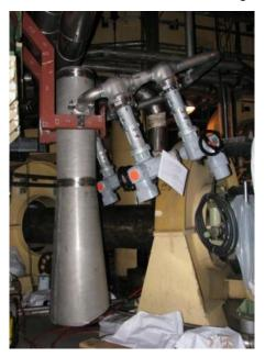
contained a separate gate valve group and a diffuser attached to the water part of each SG and allowing blowing down the secondary side of the leaking SG before having two phase or water flow through the safety valves or a water hammer. It was intended to be fully implemented on Unit No. 3 last year.
