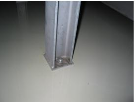
Bolted joint on the filter frame foot
