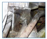
**Corrective actions**: In the future during outages of units the flanged joints connecting turbine oil system pipes and turbine bearings have to be inspected and repaired as needed.
