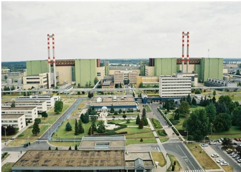
Picture 2.1-1.: View of Paks NPP (Source: www.atomeromu.hu )
