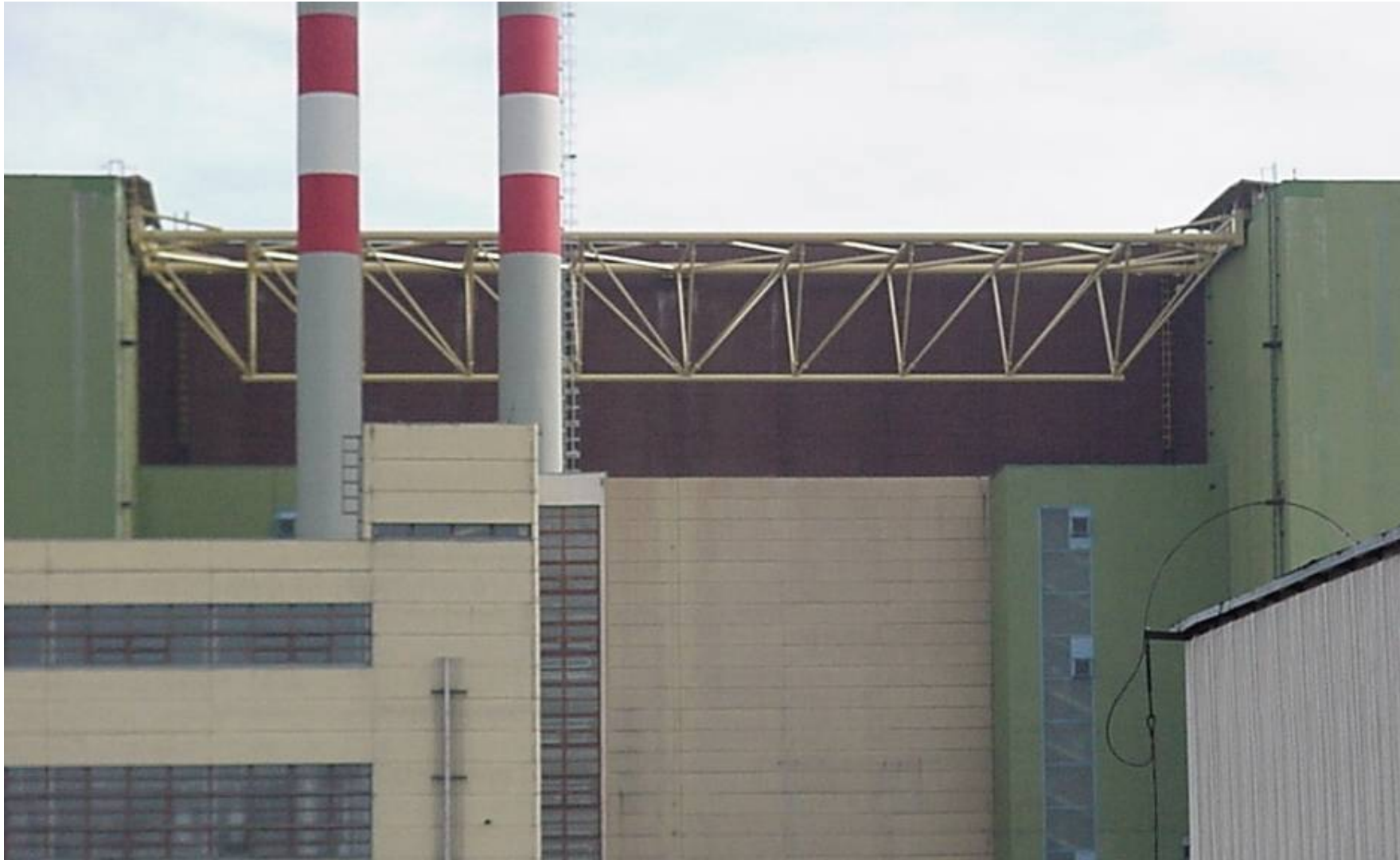
The bridge between the two localisation towers. They are also for the transfer of transversal loads to the rigid reinforced concrete part of the buildings.
