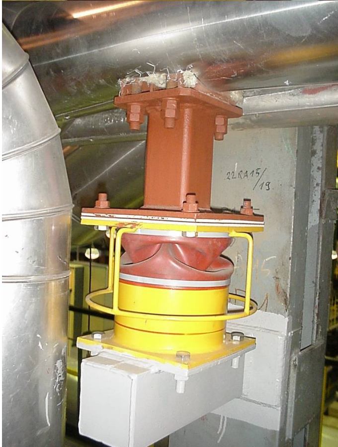
Visco-dampers on piping and equipment
