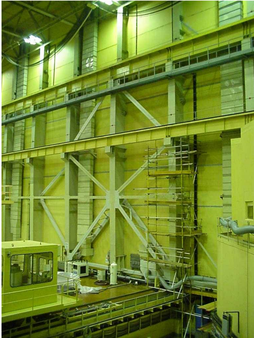
Additional X-bracing in the reactor building
