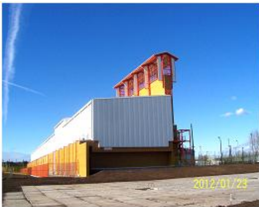
Facility extension before commissioning
