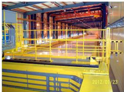
Extended charging platform
