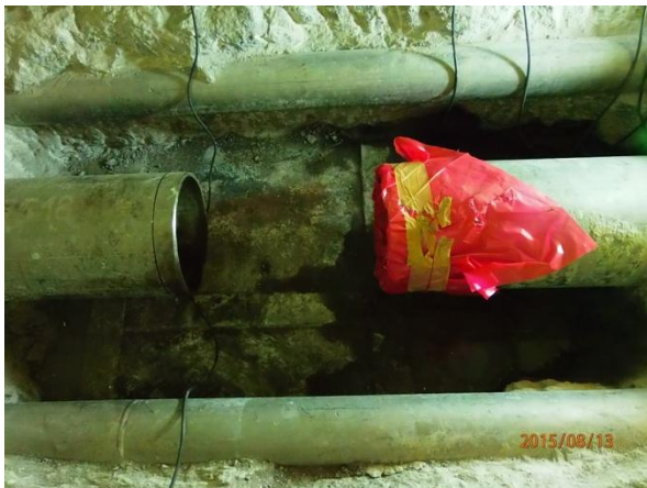
Replacement of the spent fuel pool pipeline at Unit 2
