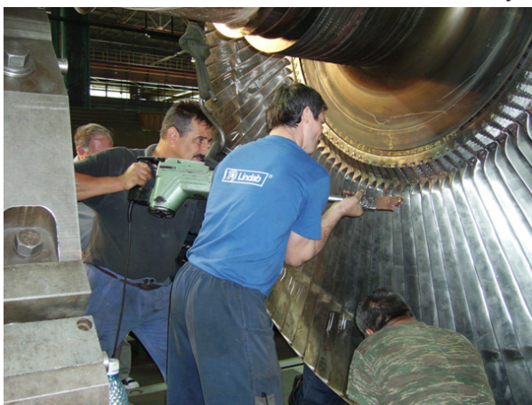
Replacement of low pressure turbine blades
