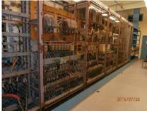
Picture 2: Safety and control rod cabinets (2)
