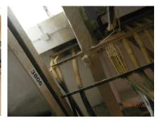
Picture 3: Fire barrier wall penetration
