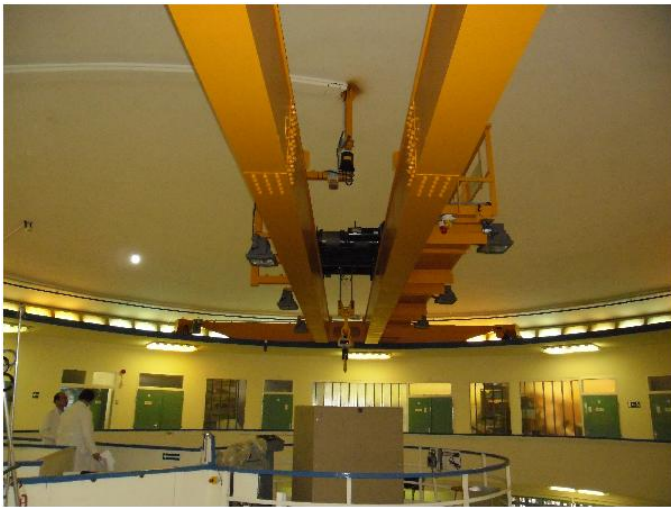
Polar crane after reconstruction
