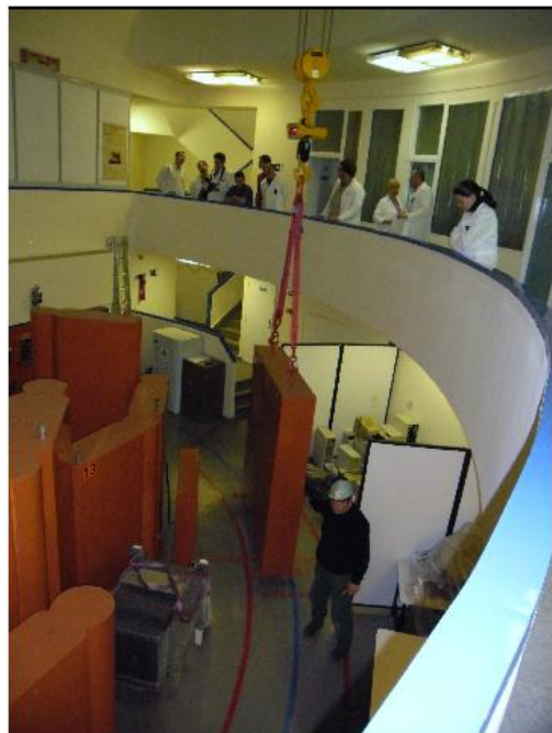
Crane load test
